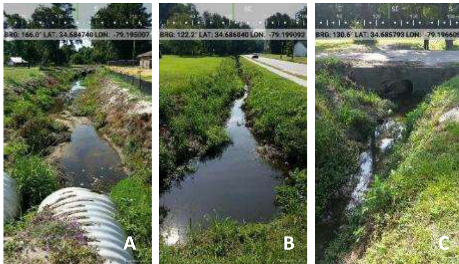
Images 4A-C. Trash, debris, and sedimentation build-up observed along short-term corridors.
