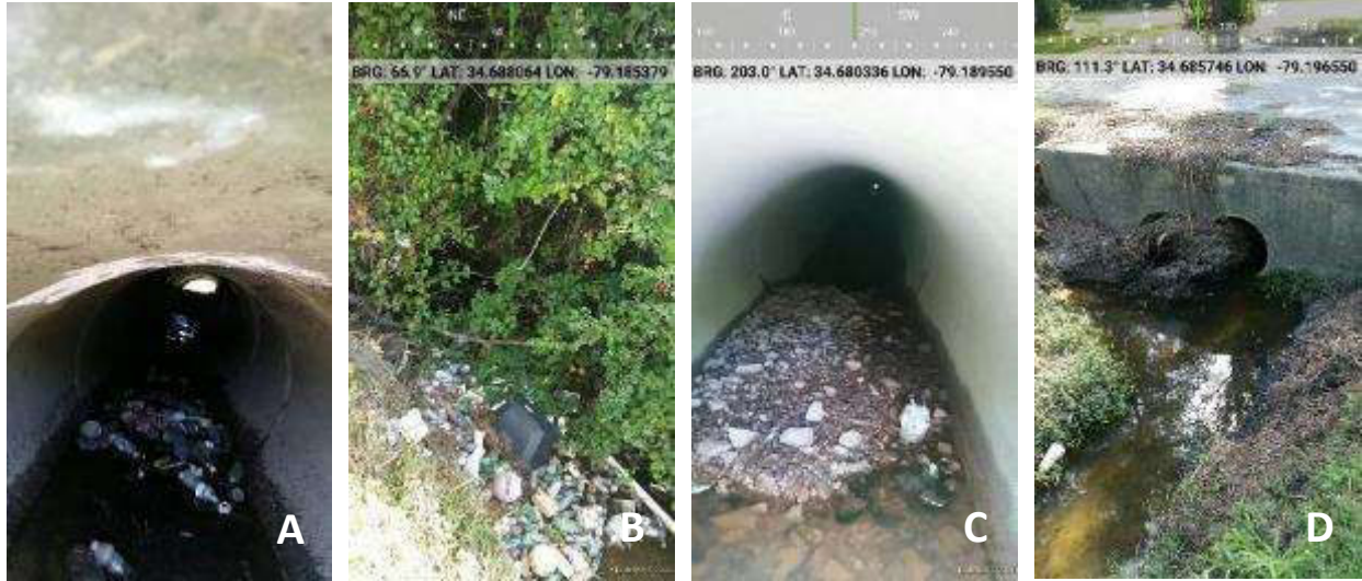
Images 3A-D. Trash, debris, and sedimentation build-up observed along short-term corridors.
